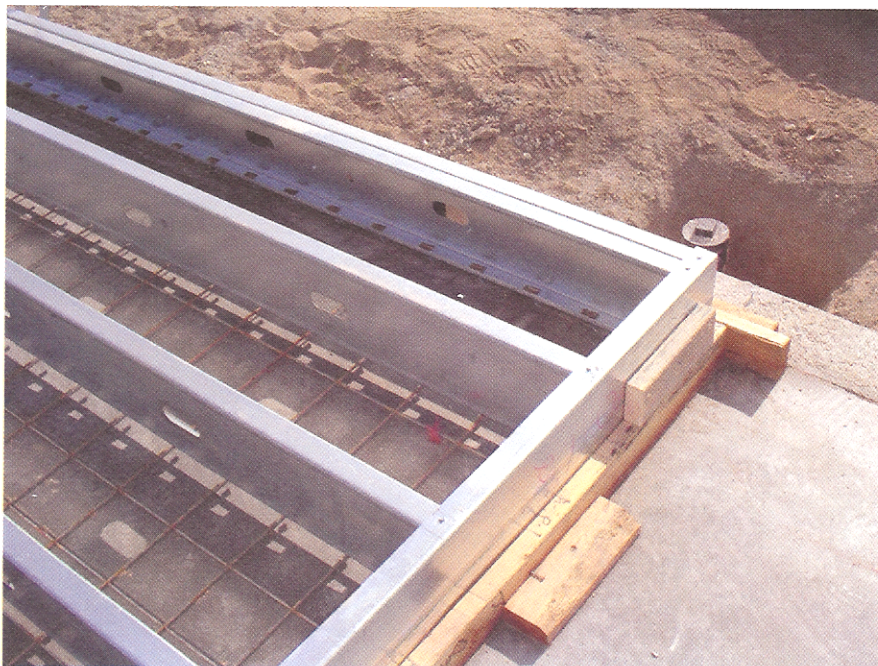
FIGURE 4 Slab used as casting surface
